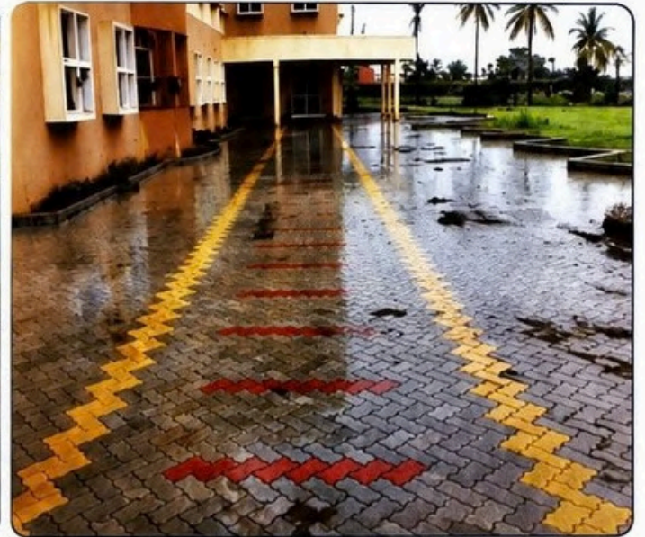
Interlocking Paver Block - Approach Road to the Building
